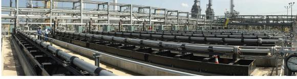
The PumpWorks HP-Plus pump was designed with reliability and cost reduction in mind. It is a multi-stage centrifugal pump capable of producing a full range of volumes and pressures. Each pump is individually assembled by trained PumpWorks personnel and fully tested to industry API 11S2 standards.
